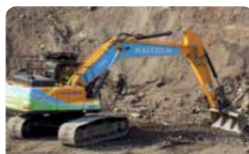
Sany SY215 22T tracked excavator
