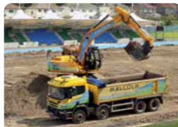
JCB JS240 24T tracked excavator
